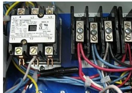
Don't forget to properly ground your control panel. Grounding is required for your protection and can save your life. There will be either a terminal block provided for ground wire connection OR a loose wire may be provided for grounding to your input power with a wire nut or crimp connector.
